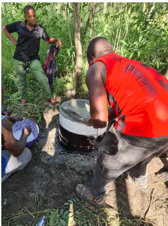
Figure 1. VLFR boundary consolidation by using Laqiline drums filled with concrete mixture as permanent marks.
