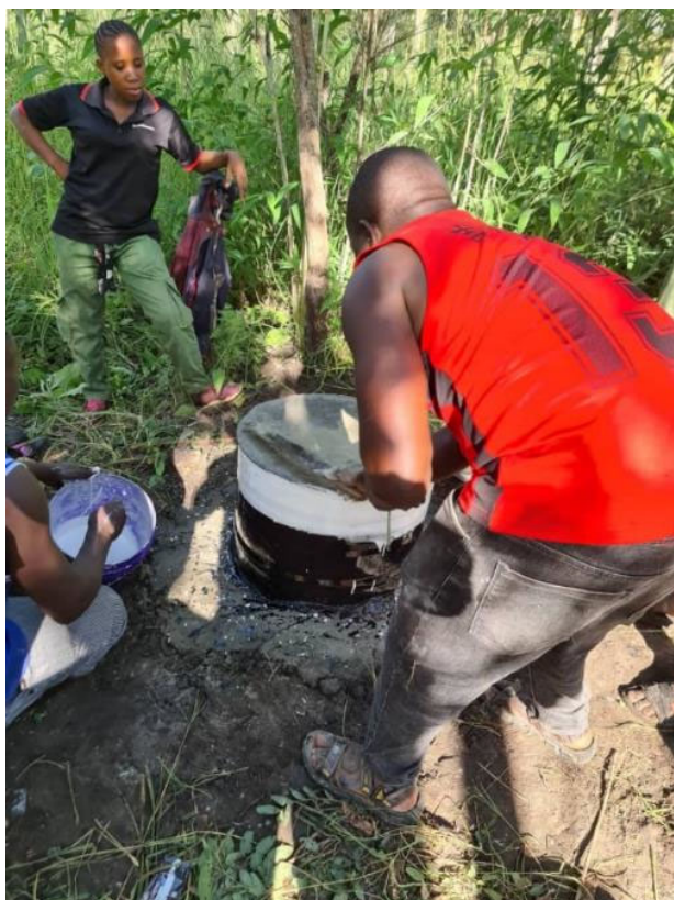
Figure 2. VLFR boundary consolidation by using Laqiline drums filled with concrete mixture as permanent marks.
